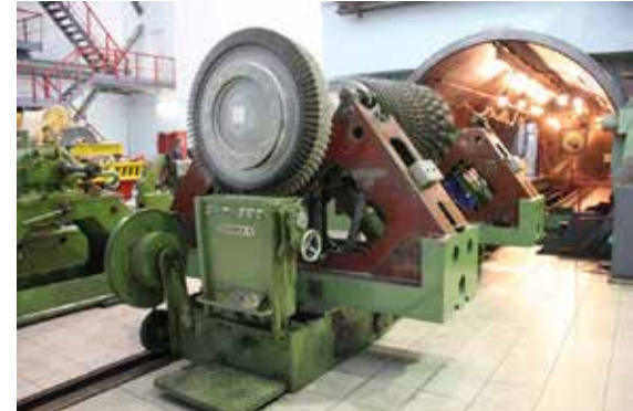
Shenk high-speed balancing and overspeed facility
