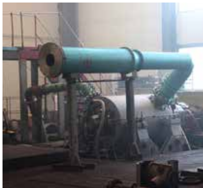
Replaceable Flow Passage 155-1076-2.2C for the booster compressor station of OOO Gazprom Dobycha Urengoy
