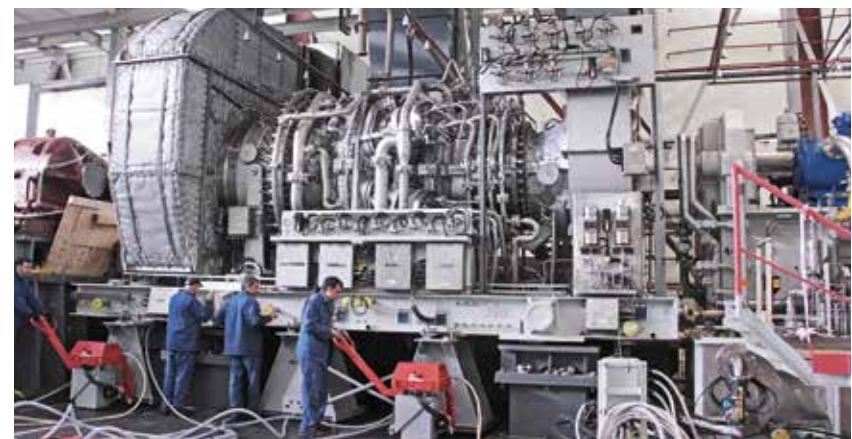
Installation of T32 GTU on the test bed of Nevskiy Zavod manufacturing site
