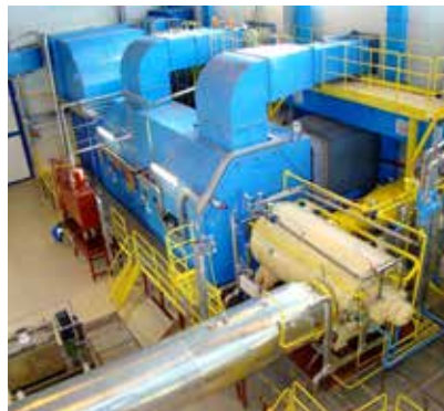
295 Replaceable Flow Passage at the booster compressor station of Zapadno-Tarkosalin gas field of OOO Gazprom Dobycha Noyabrsk
