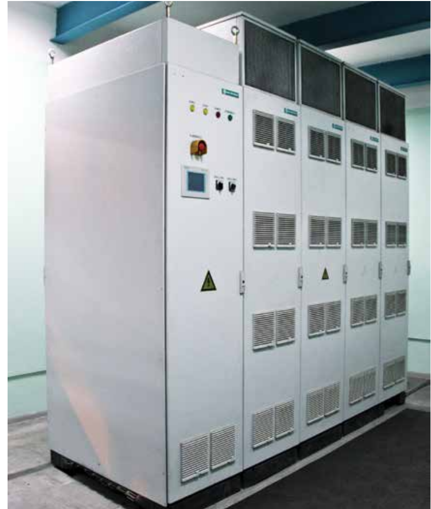
Frequency converter ПЧТ-6-2600-B-01
