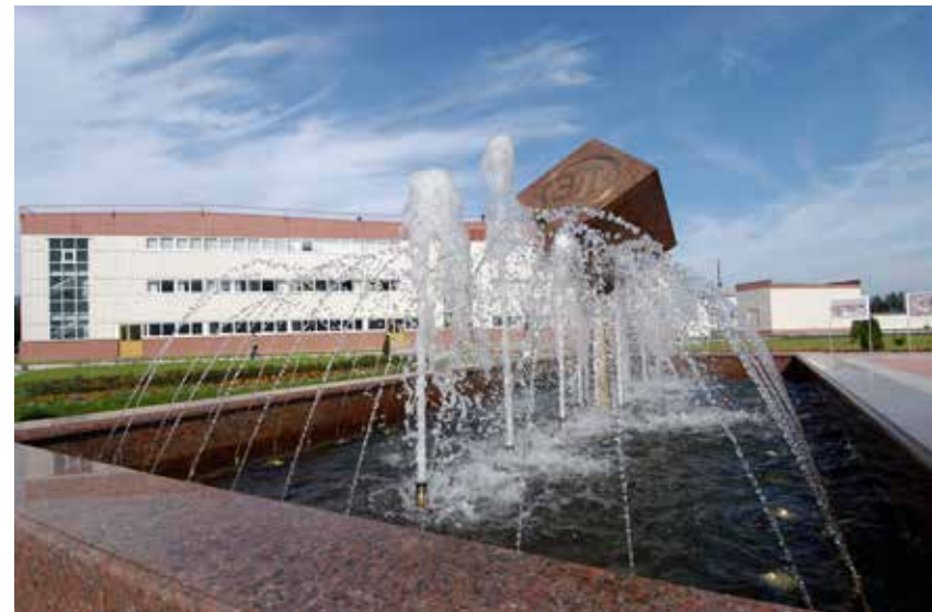
Production site “ELECTROPULT Plant”, Electrical Equipment Complex
