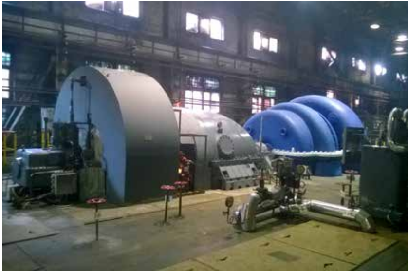
Turbocompressor Unit 5200/25 at Magnitogorsk Iron & Steel Works
