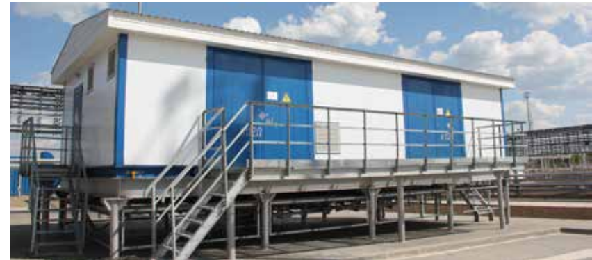
Control Rooms at CS-8 "Chikshinskaya"
