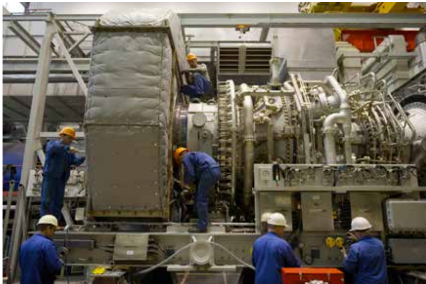
Installation of GTU-32 on the test bed of Nevskiy Zavod
